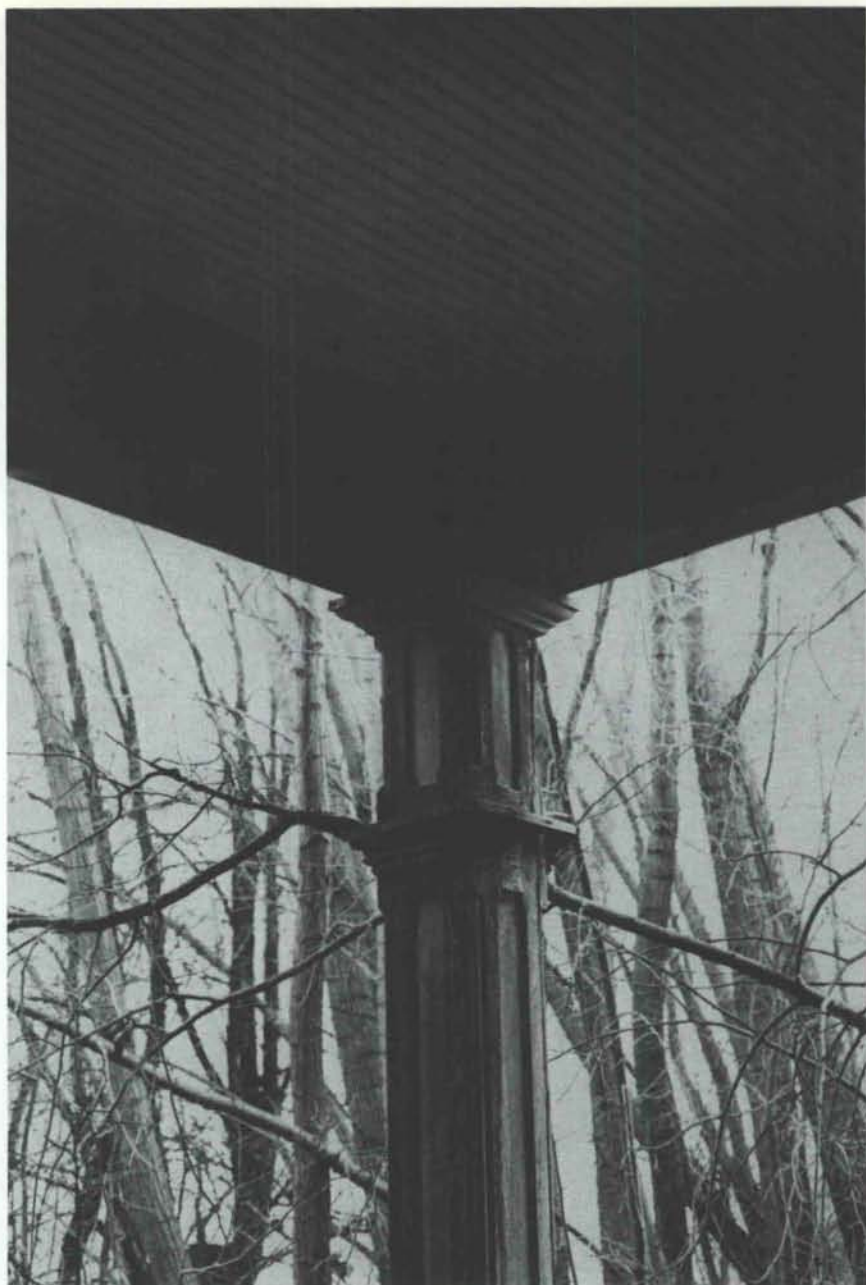
Column at front porch. Folk version of the Territorial style based on the Greek revival.
