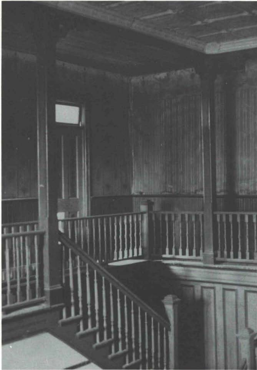
A stairway of two runs ascends to the second floor. The balcony runs all four sides of the stair and open well over the main hall.
